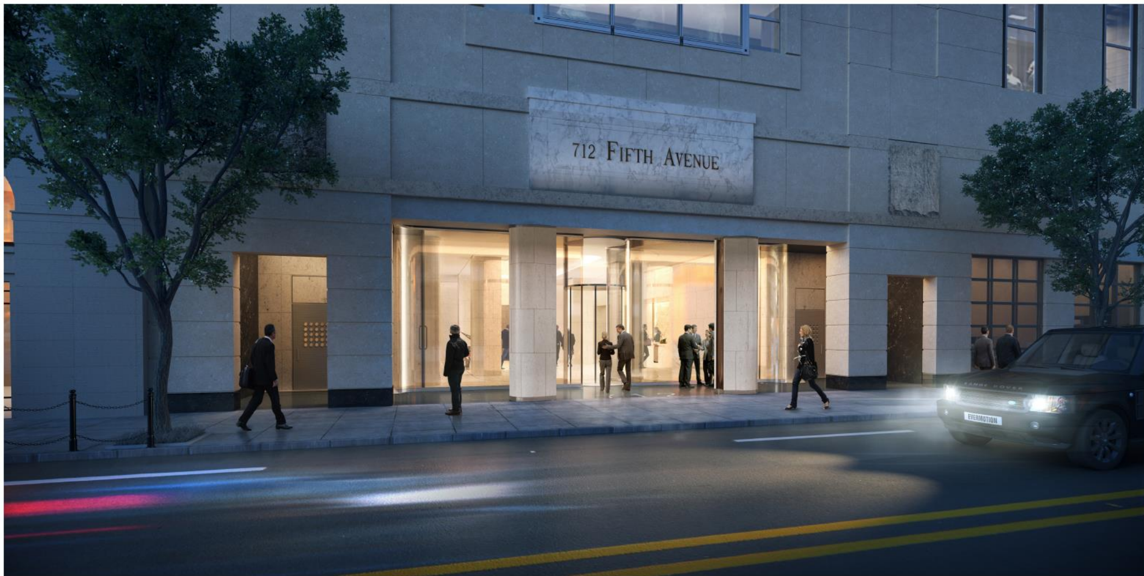
LOBBY ENTRY WITH NEW COLUMNS
