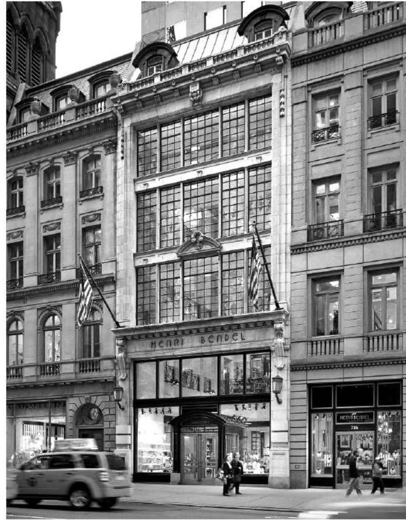
HENRI BENDEL AT FIFTH AVENUE
